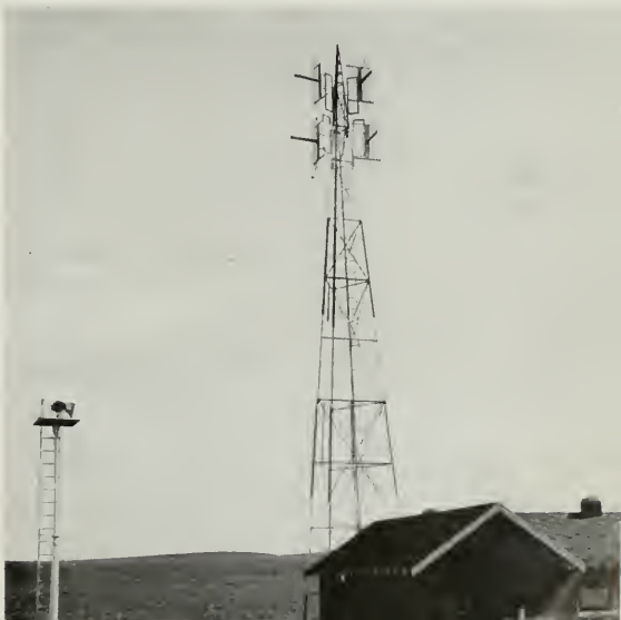
This tower near Calgary supports radio antennas which feed signals north and west of the Canadian city.
