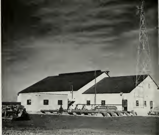
This microwave station at Edmonton, operated by Northwestern Utilities, serves as communications center for 40 mobile vehicles.
